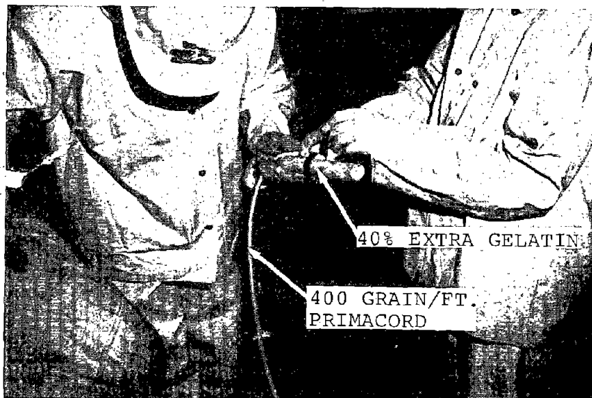
FIGURE 4-5. PRIMACORD PERIMETER HOLE LOADING (WITHOUT SPIDER TUBE)
