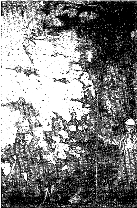
(a) Left Rib, Notched Perimeter Holes (b) Right Rib, MSB Space Loading
