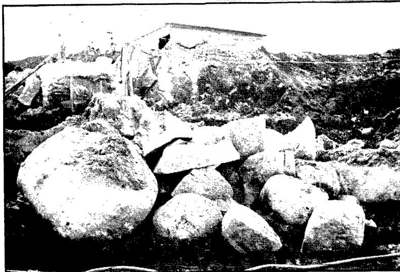
Massive boulders requiring special rotary-type equipment.▼
