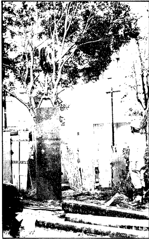
FIGURE 9 EXTRACTION OF STOP END PIPE
