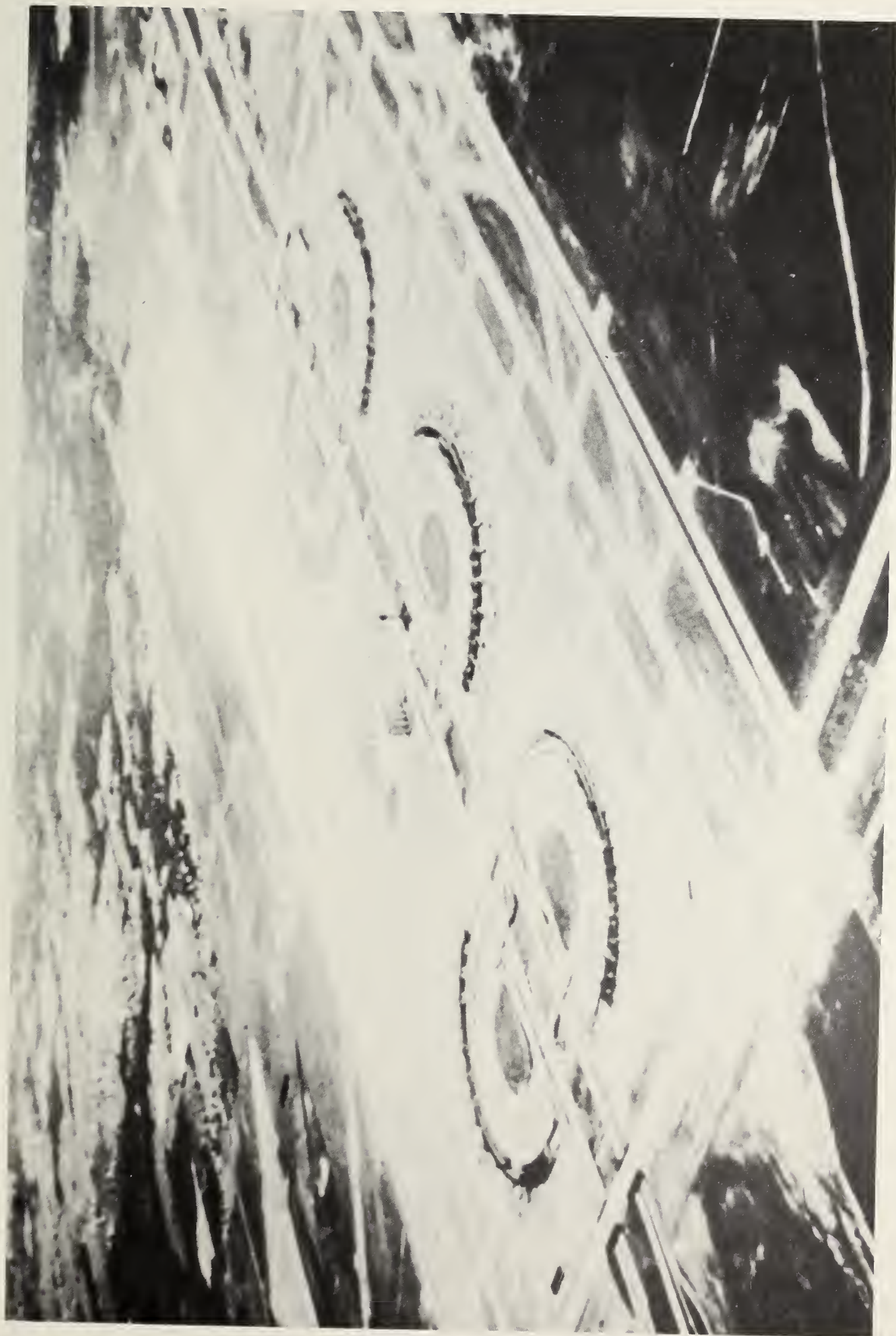
FIGURE 1-5. AN AERIAL VIEW OF THE DALLAS-FORT WORTH AIRPORT
