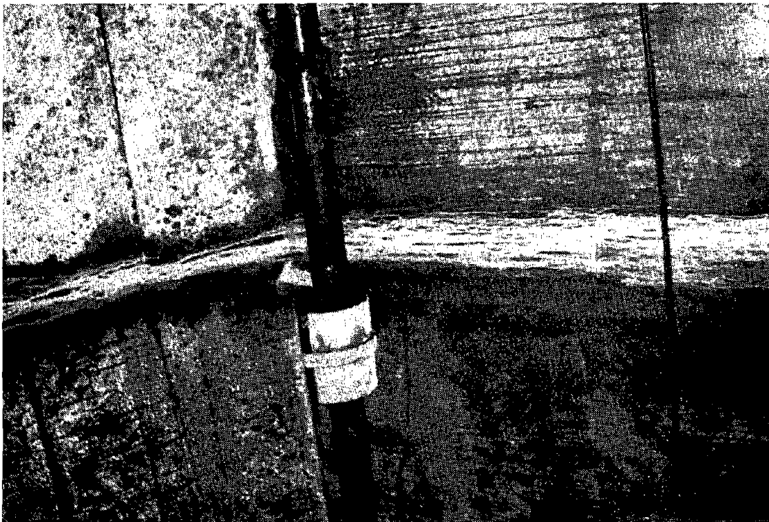
FIGURE 9.16 WATER INFILTRATION THROUGH CONSTRUCTION JOINTS
