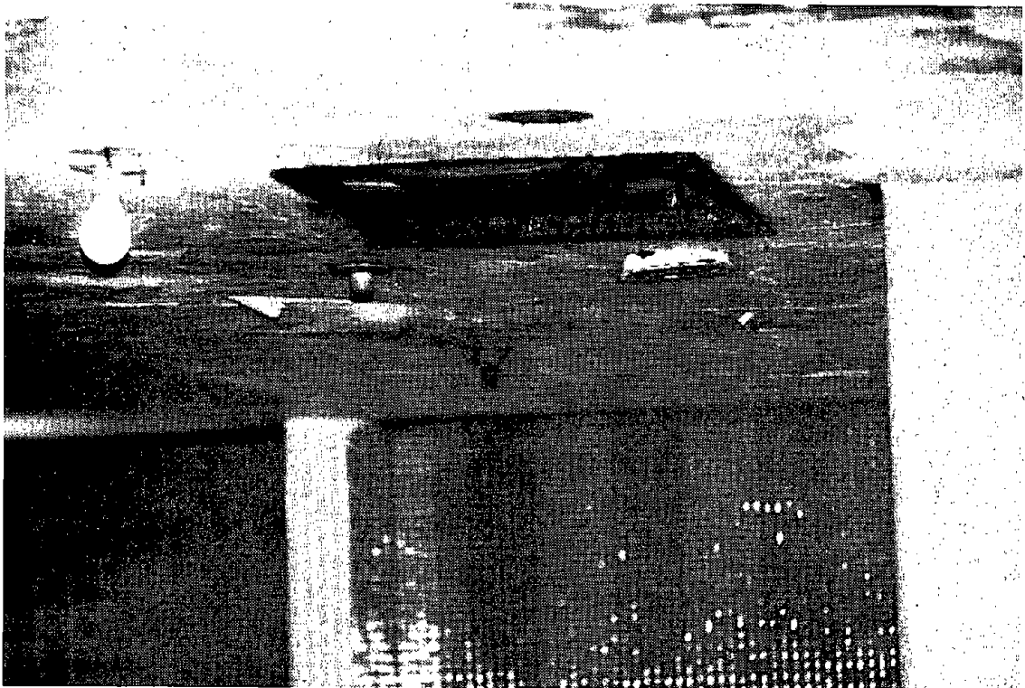
FIGURE 7.9 CEILING SECTION REMOVED FOR INVESTIGATION OF MAIN ROOF LEAKS (BLUE LINE, AQUARIUM STATION)
