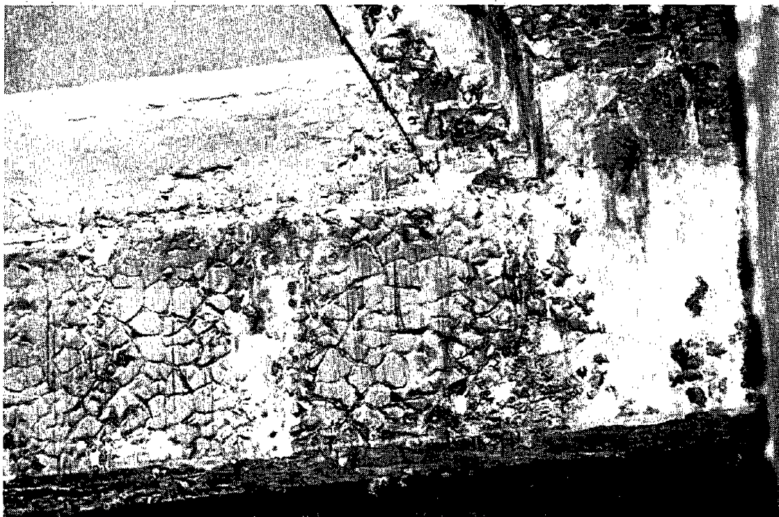
FIGURE 7.10 CALCIFICATION OF THE WALL FINISH (BLUE LINE, AQUARIUM STATION)
