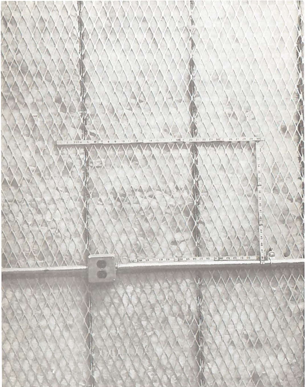
Figure 4. View of Interior Cell Wall "Soft Lining"
