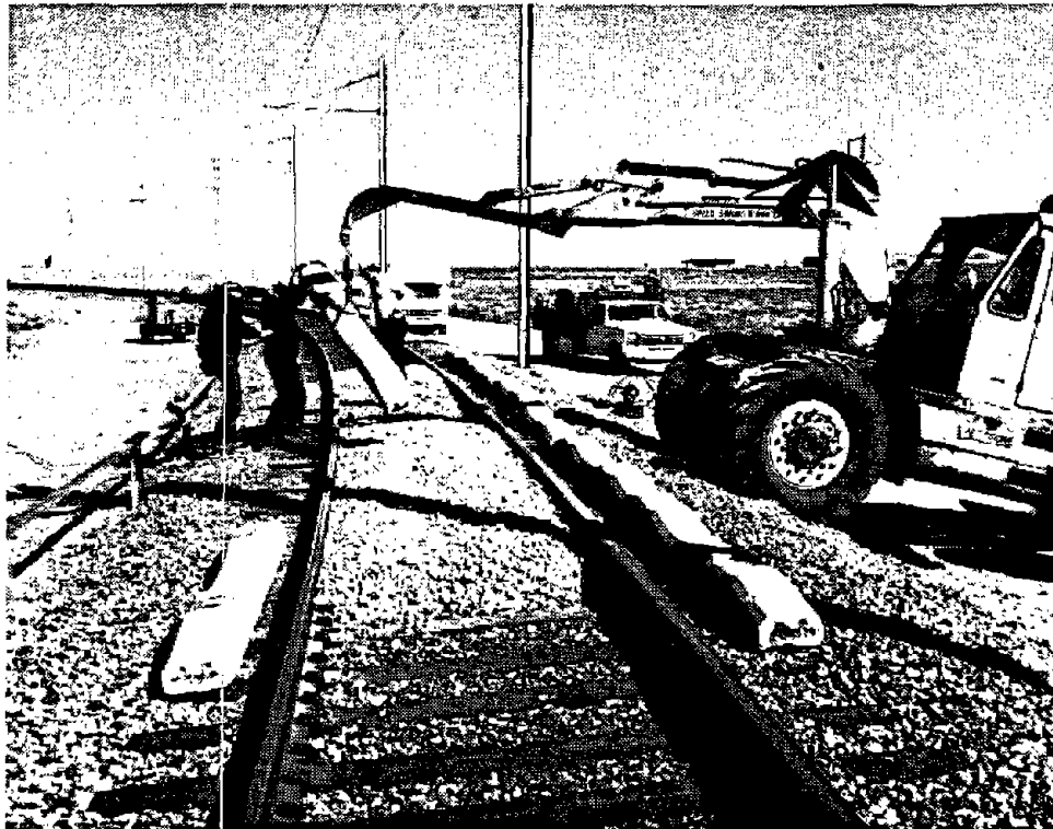
FIGURE A-5. ADDITIONAL STIFFENING FOR THE STATIC BUCKLED ZONE (CONCRETE TIES PLACED AT ENDS TO INCREASE WOOD TIE-BALLAST FRICTION)
