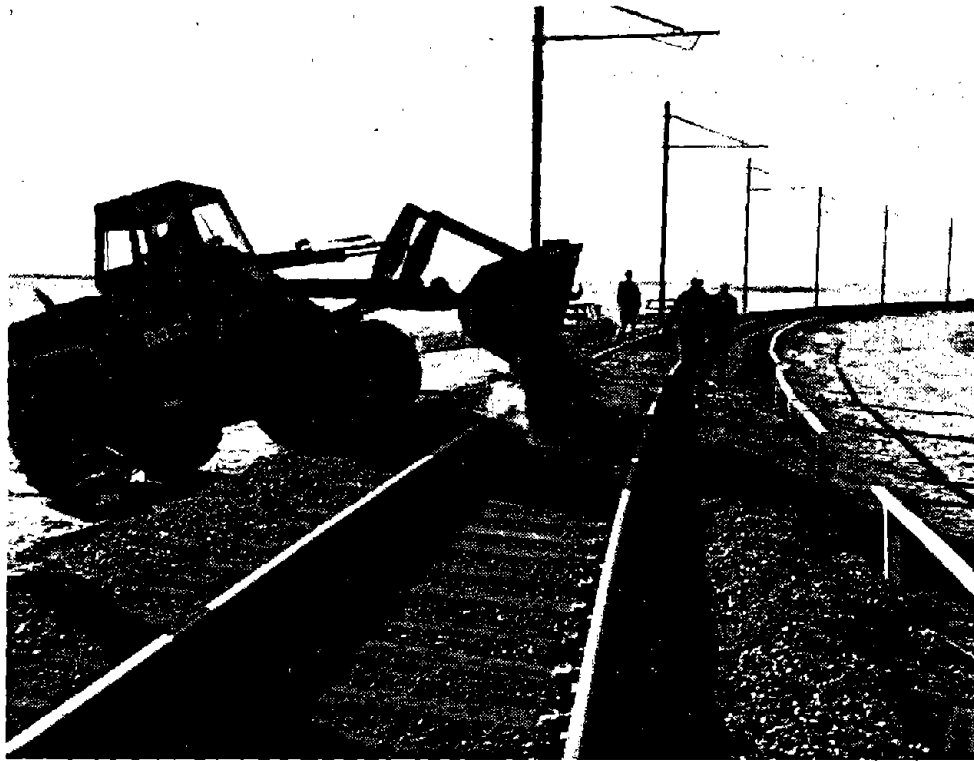
FIGURE A-3. BALLAST ADDITION TO REINFORCE TRACK BUCKLED IN STATIC TEST
