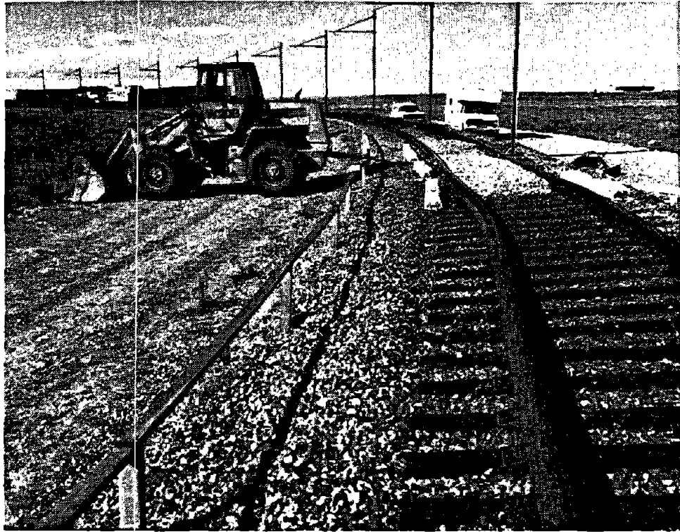
FIGURE A-9. DYNAMIC BUCKLE NEAR LOCATION 6
