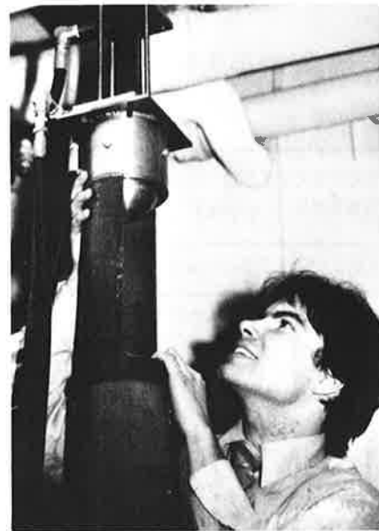
(B) Mounting projectile in grip collar.
