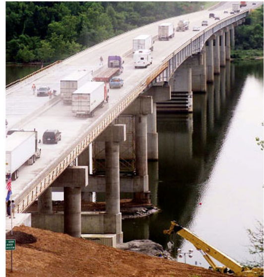
Figure 9 New I-40 Bridge
