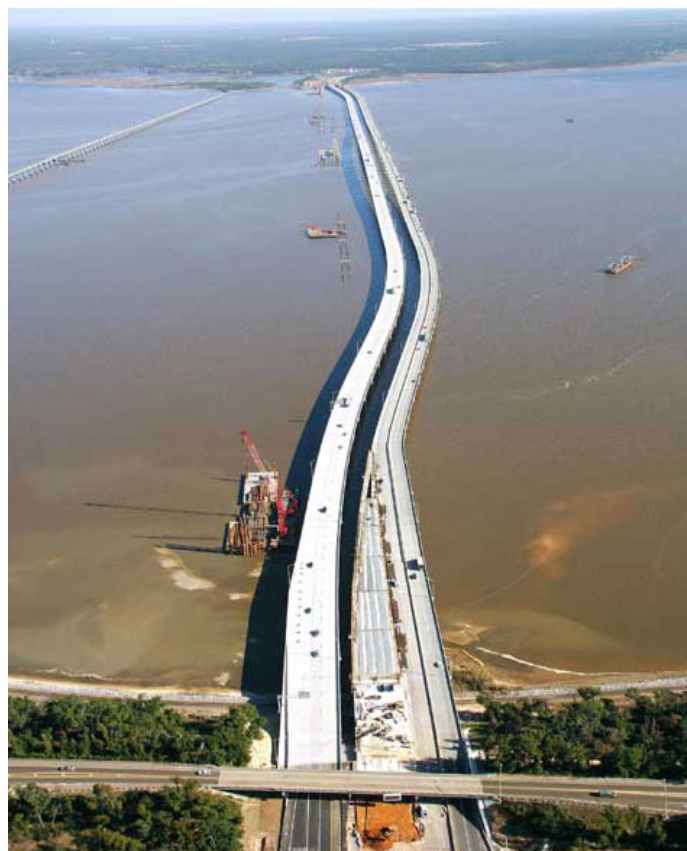
Figure 4 New I-10 Bridge
