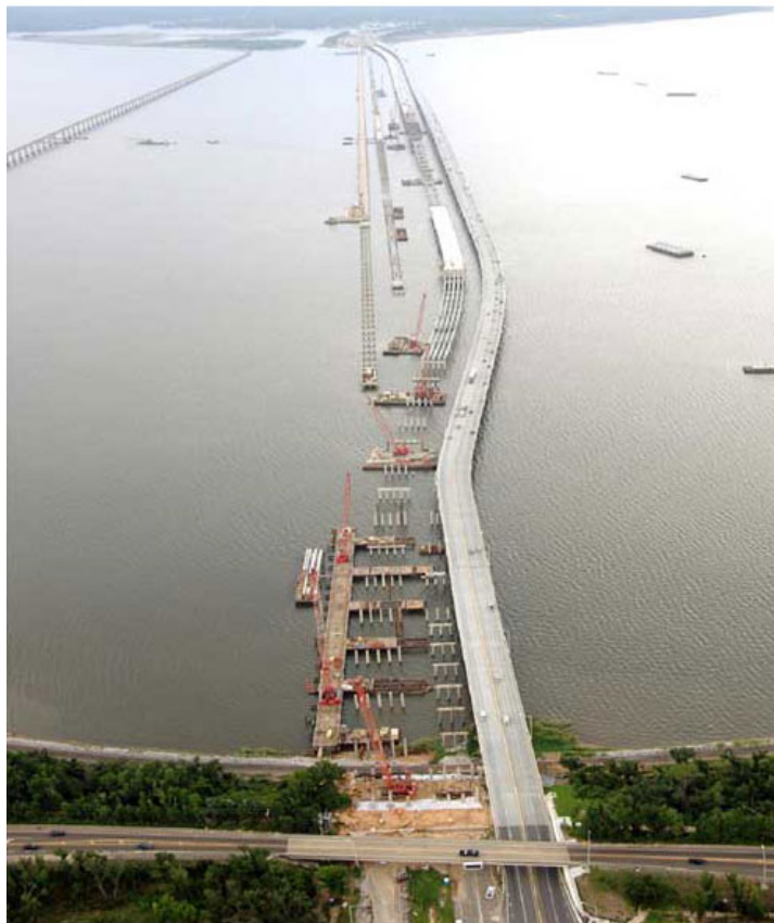
Figure 3 I-10 Bridge Reconstruction
