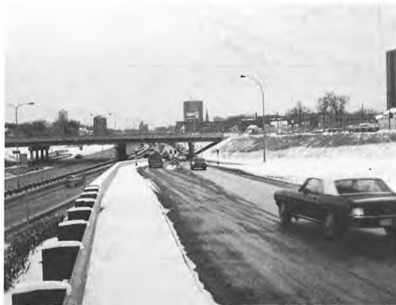
Figure B-1. Ramp Meters and Bypass Lane for Buses, I-35W, Minneapolis, Minnesota
