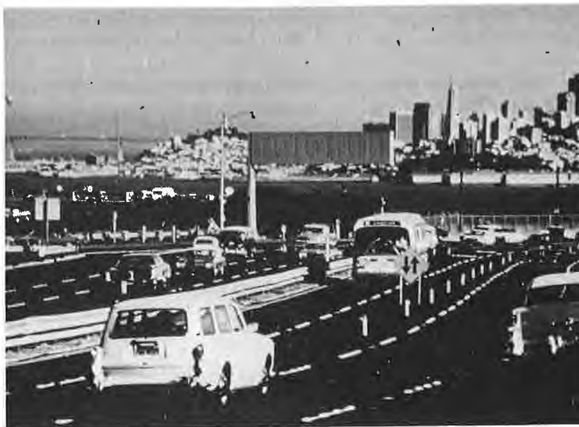
Figure 10. Contraflow Bus Lane - U.S. 101, Marin County, California
