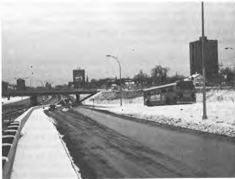
Figure 8. Minneapolis I-35W: Metered Ramp with Bypass Lane for Express Buses
