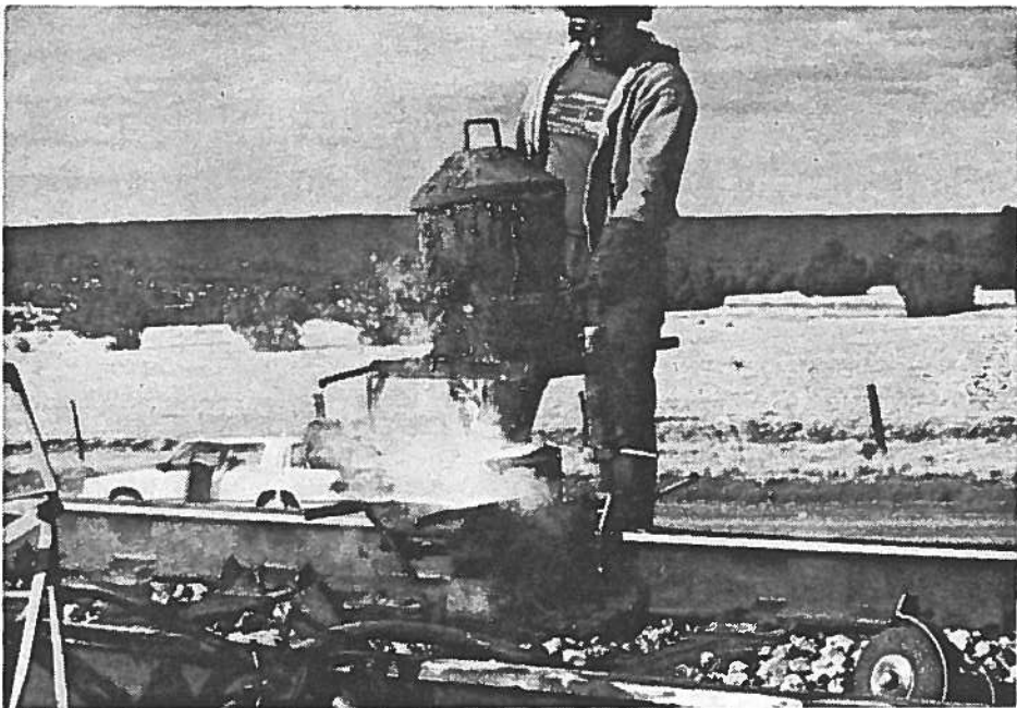
Figure C-8. Welding the High Rail in TS1
