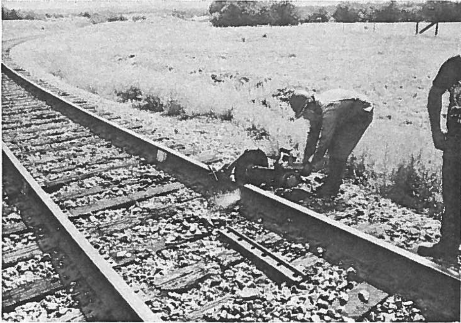
Figure C-7. Cutting the Low Rail in TS3
