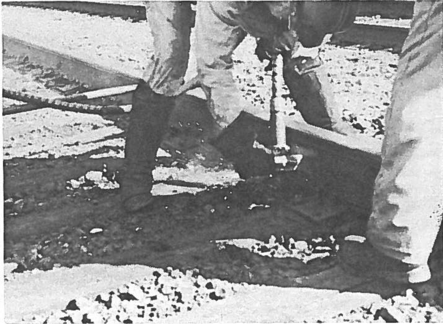
Figure D-1. Rough Grinding of Rail for Strain Gauge Application
