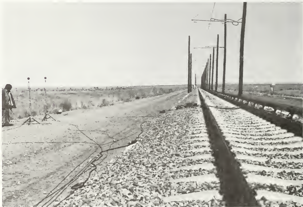
(b) Welded Rail on Concrete Ties.
