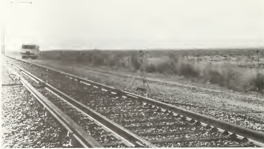
(a) Jointed Rail on Wood Ties.
