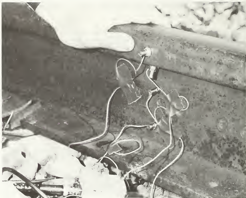
FIG. 63. RAIL ACCELEROMETER LOCATIONS (TTC PHOTO).
