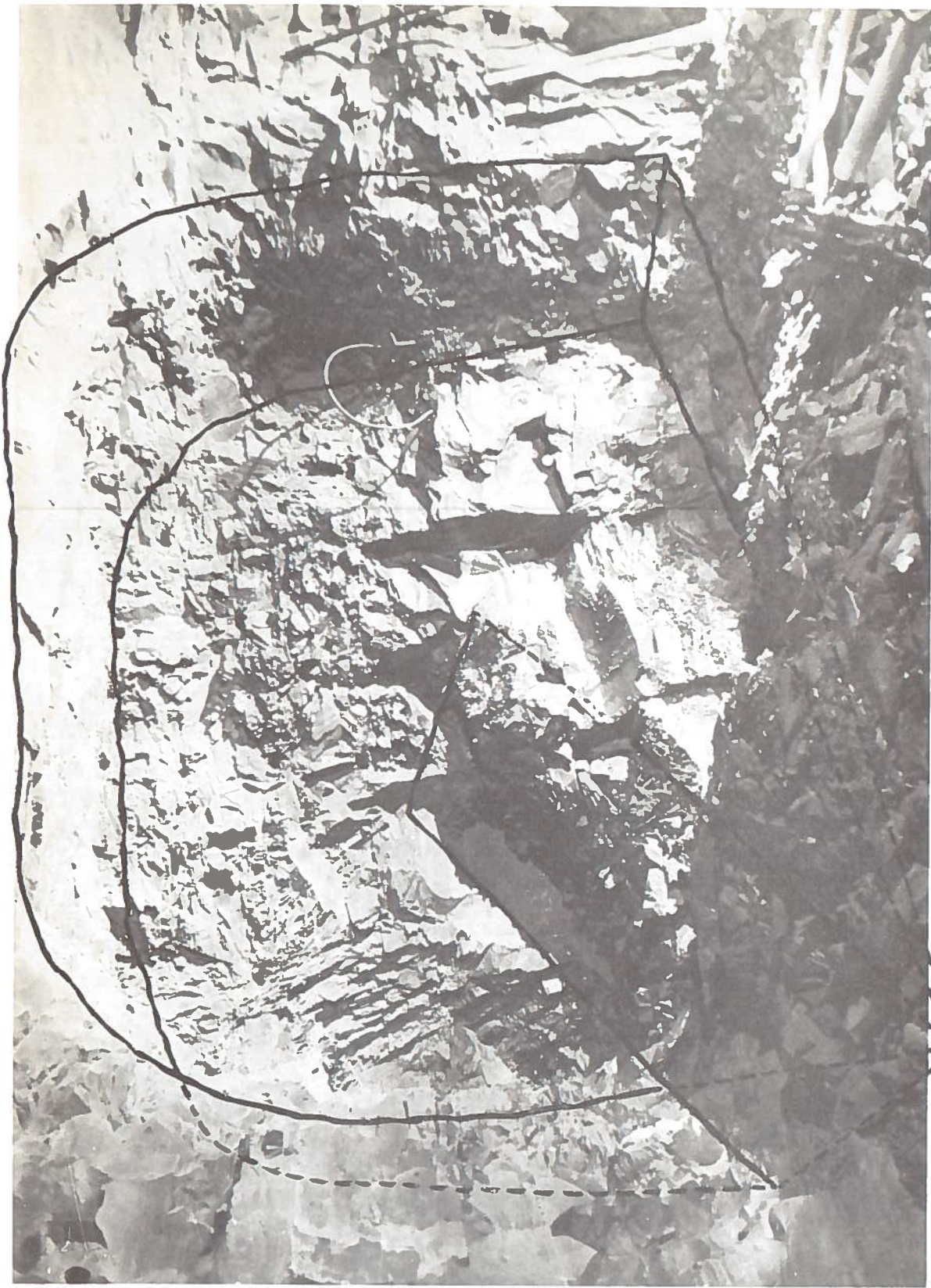
FIGURE 8 SPIRAL BLAST CONFIGURATION, LEFT QUARTERING VIEW SHOWING "IDEAL" GEOMETRY
