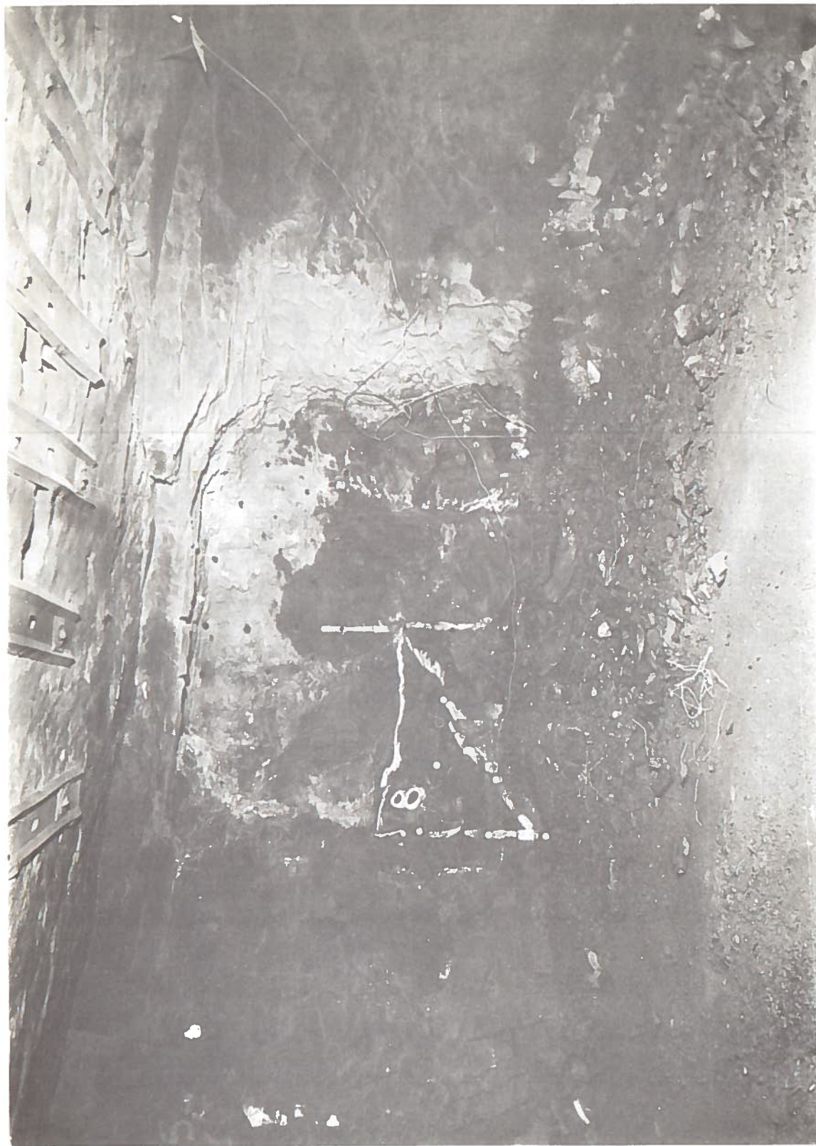
FIGURE 6 SPIRAL BLAST CONFIGURATION, HEAD-ON VIEW
