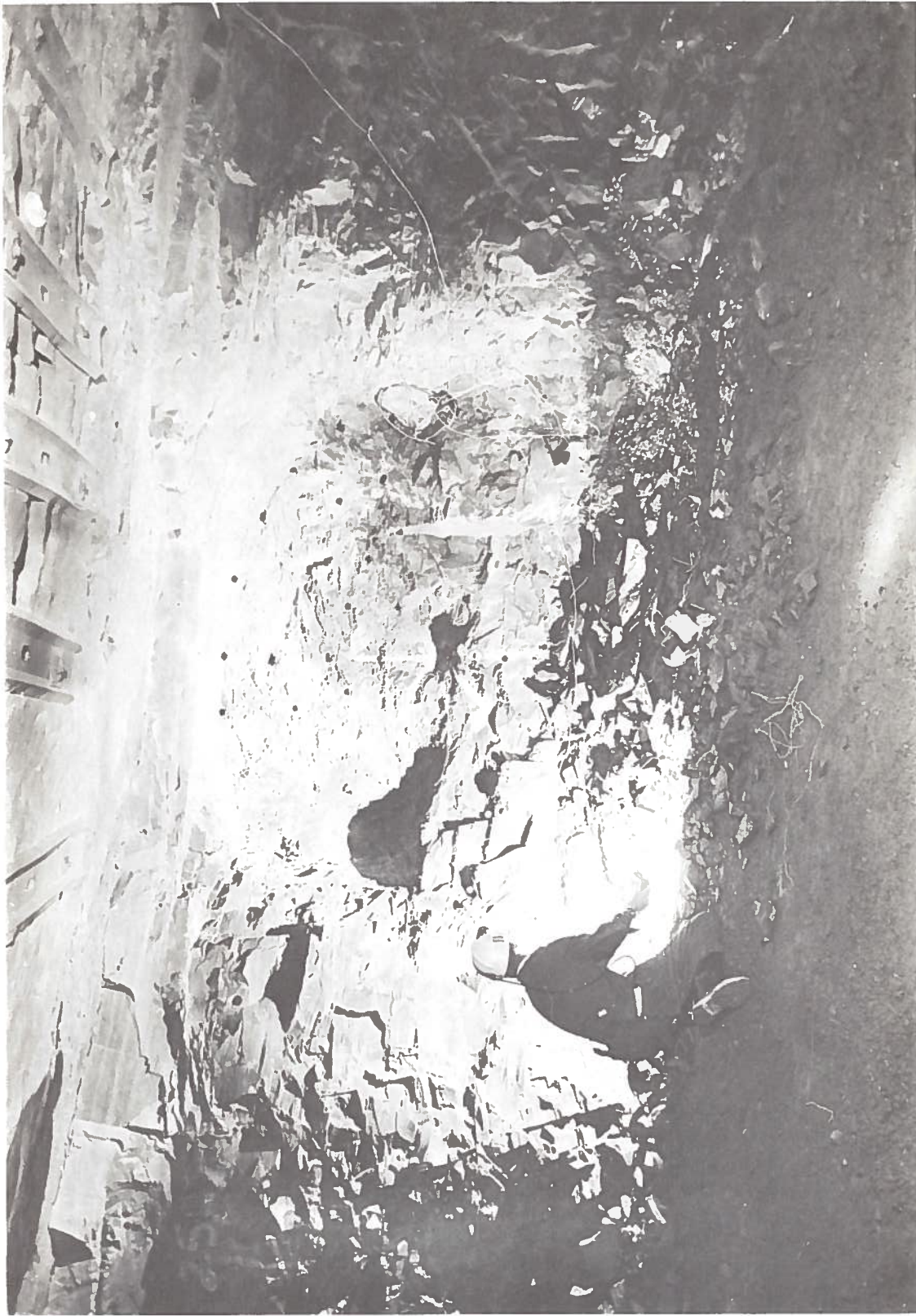
FIGURE 7 SPIRAL BLAST CONFIGURATION, HEAD-ON VIEW
