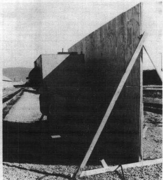
FIG. 4. CONFORMING SITE (SITE NO. 2) LOAD CELL INSTALLATION WITH BARRIER
