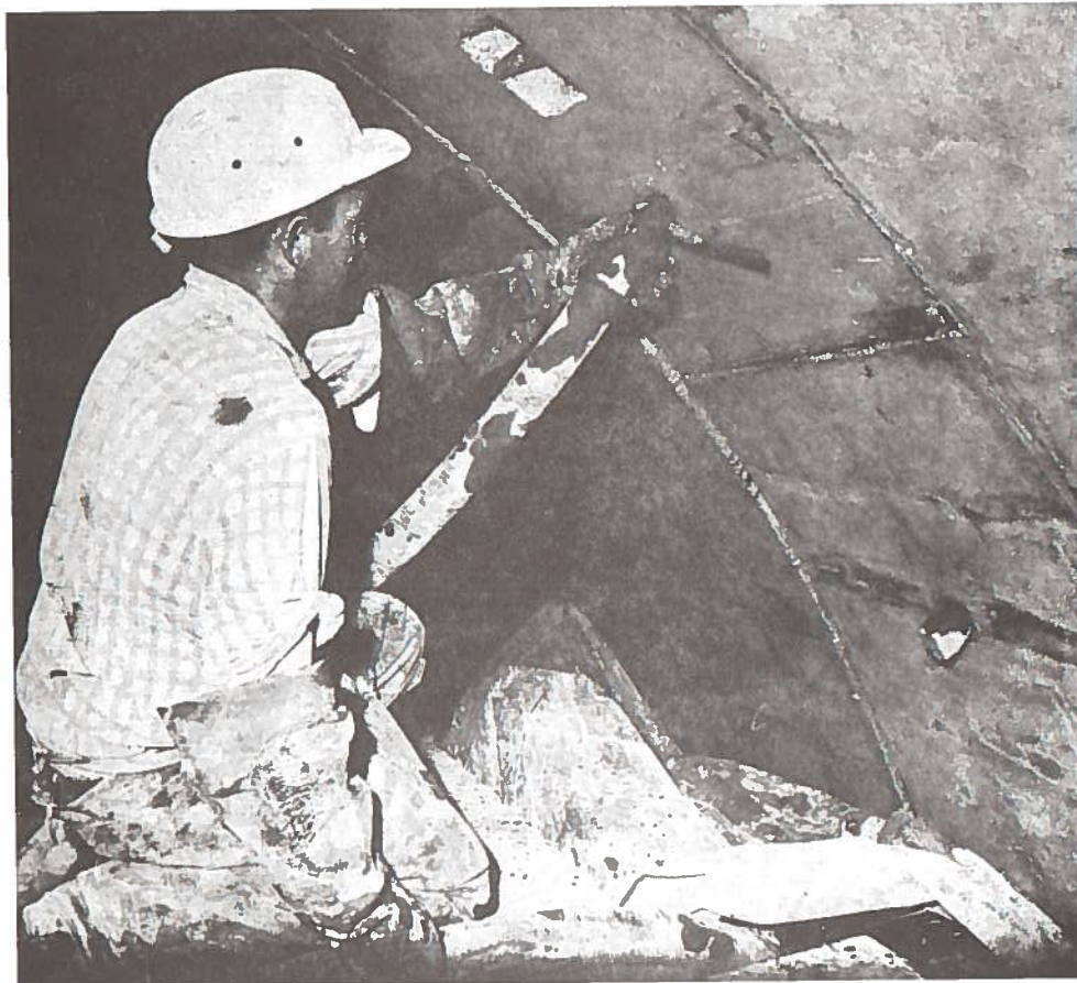
Grouting of the cavity between lining and ground
