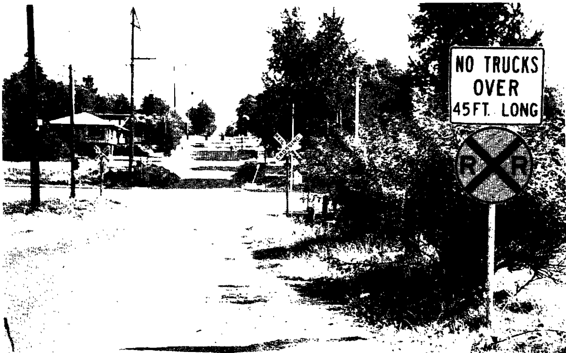
FIGURE 3-4 Crossings Scheduled for Improvement in Oregon Involve Installation of Gates Coordinated with Traffic Signals
