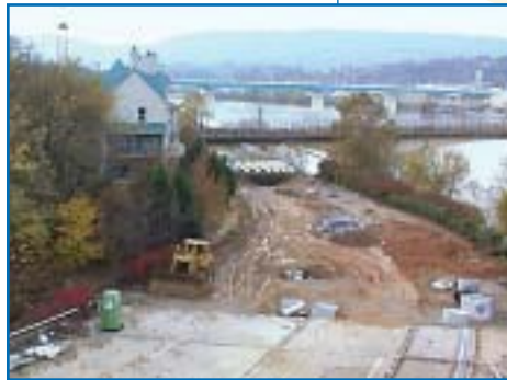
The Riverfront Parkway is being reduced from an expressway to a livable street in Chattanooga.
