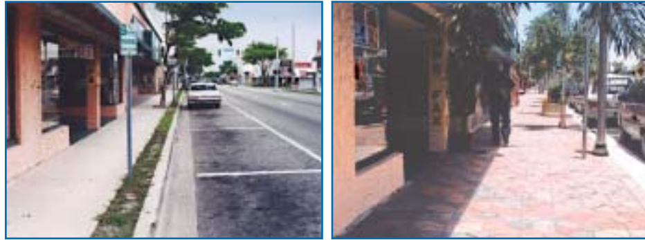
Street reconstruction in Delray Beach before and after.
