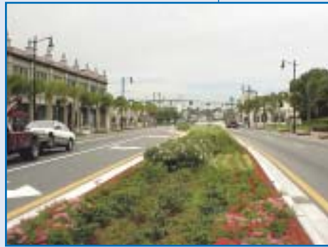
The final construction of the landscaped median on U.S. Route 1 would have been nearly impossible without the cooperation between FDOT and the city of Fort Pierce.
