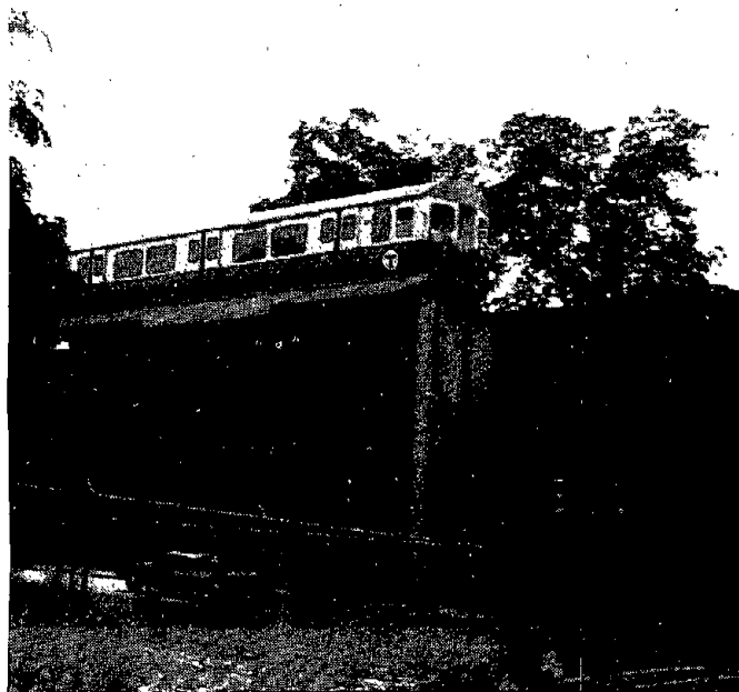
FIGURE F-4. ORANGE LINE ELEVATED STRUCTURE WITH LATTICE WEB GIRDERS
