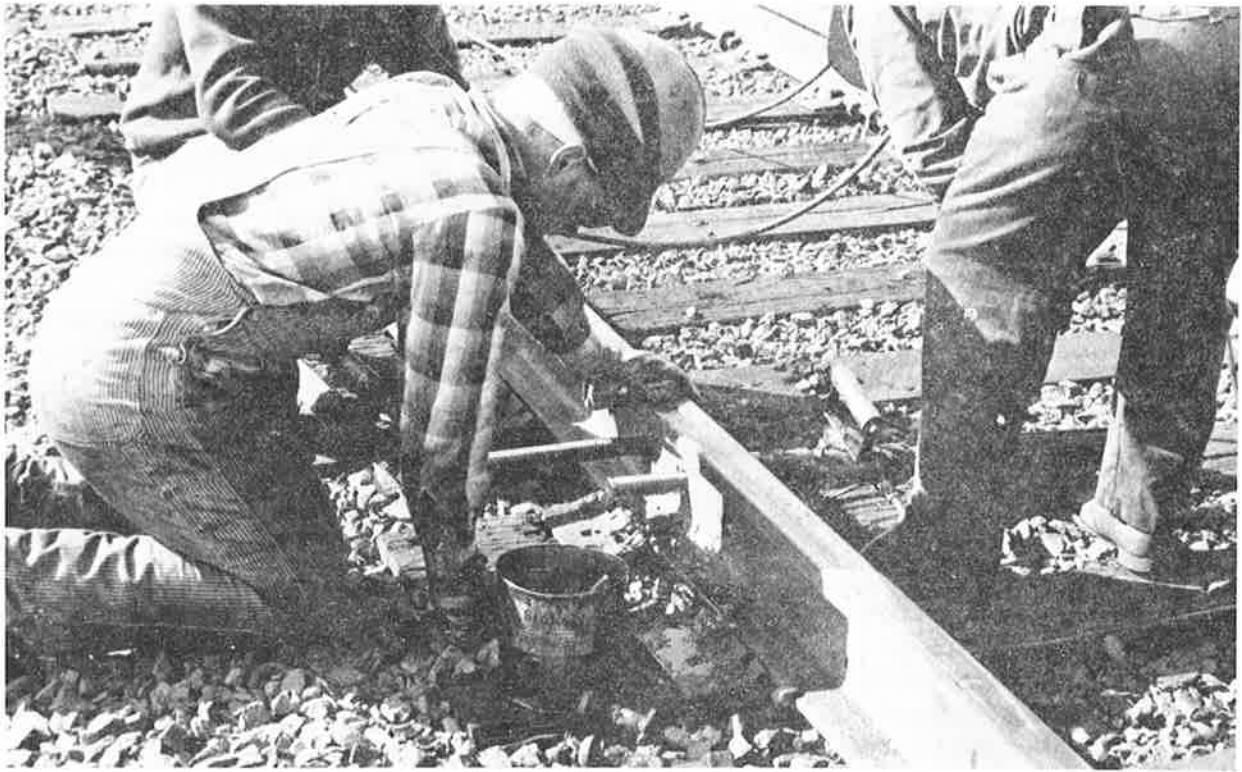
Figure 36.—Broaching Track Joint Holes in the Field
