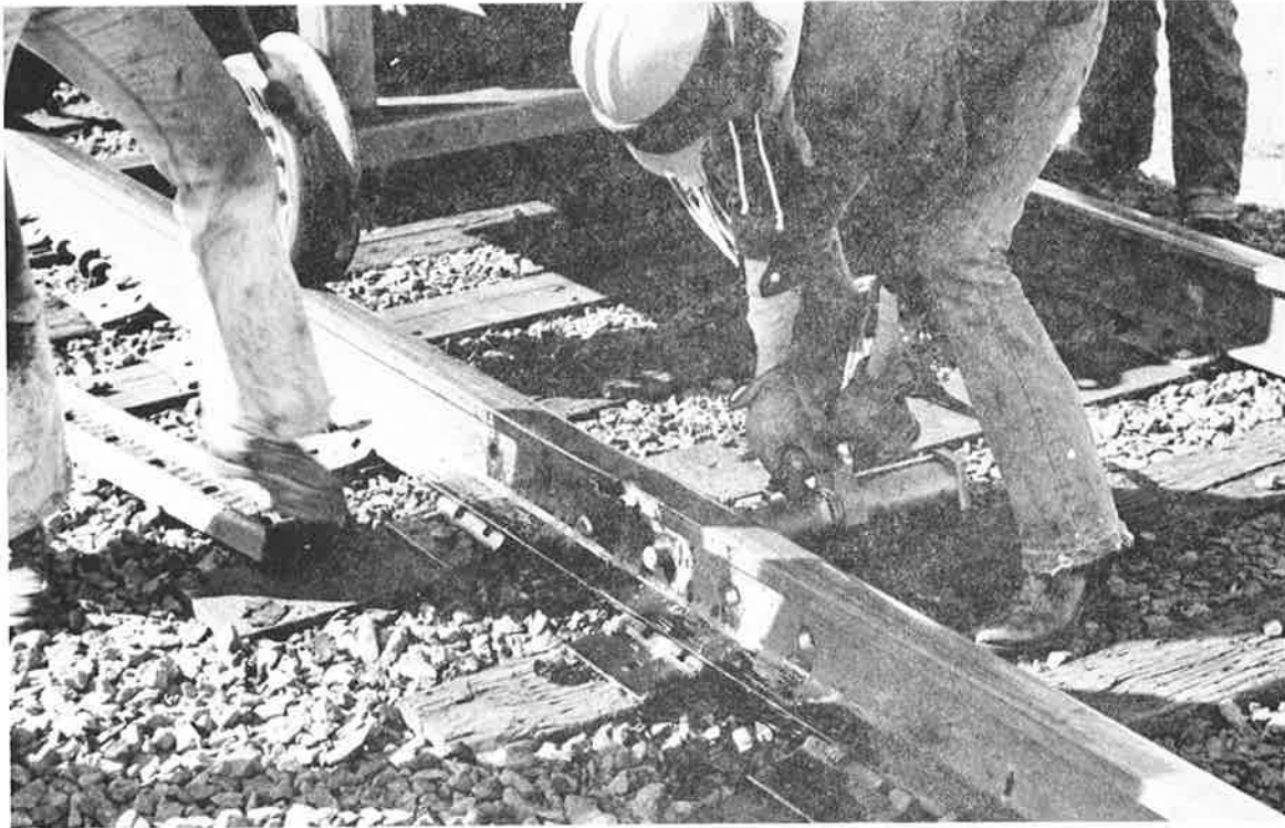
Figure 38.—Cold Expanding Joint Holes in the Field
