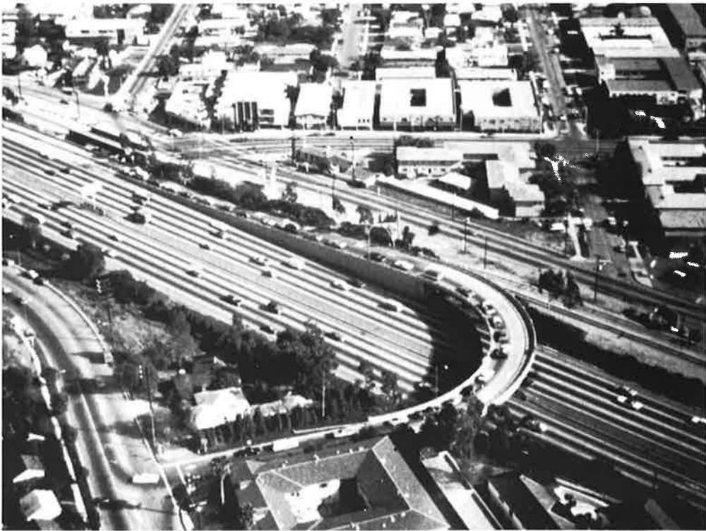
Autos Waiting at Metered On-ramp with Bypass Lane for Buses and Carpools, Santa Monica Freeway, California
