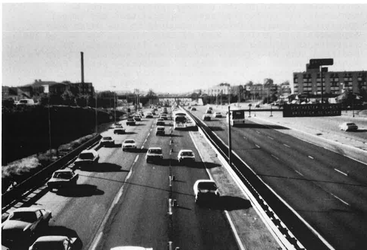
Reserved Bus and Carpool Lane, Southeast Expressway, Boston, Massachusetts
