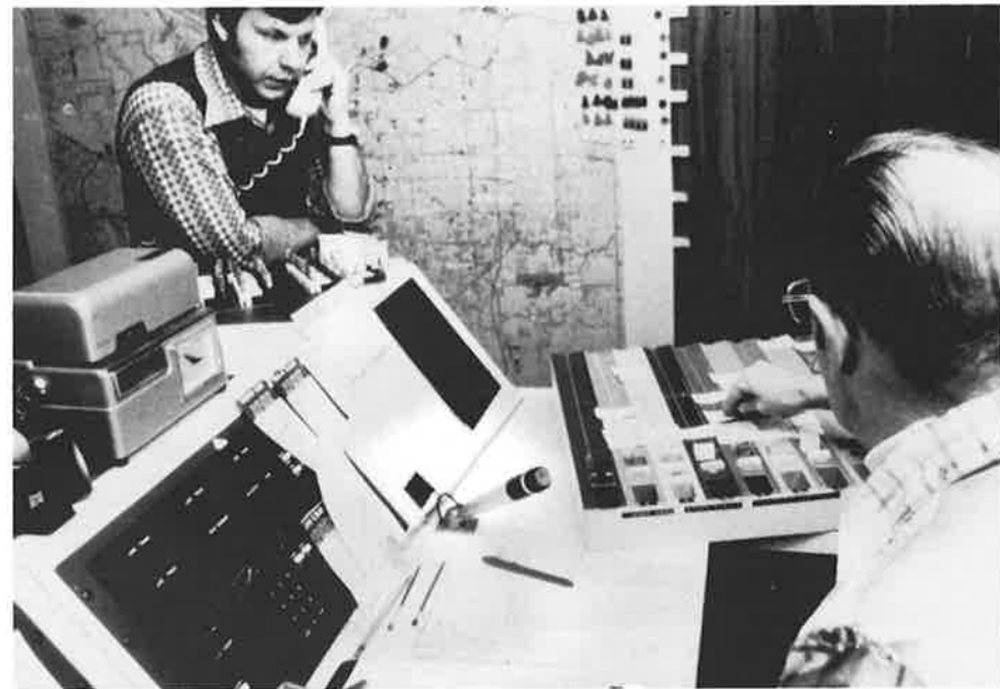
Control Center, Portland, Oregon
