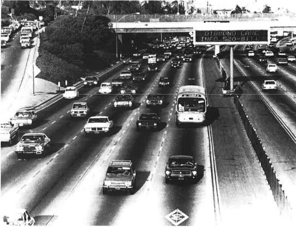
Diamond Lane in Operation Showing Electronic Sign and Autos Waiting at Metered On-Ramp, Santa Monica, California
