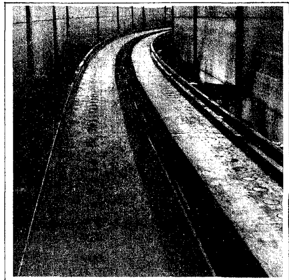
Figure 2-9. Installed Surfaces Looking South
