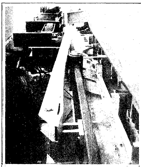
Figure 2-21. Switch Arm Moving Switch Wheels
