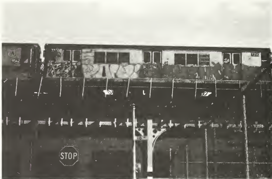
FIG. C.1. NYCTA ELEVATED STRUCTURE AT 10th AVENUE AND 207th STREET.
