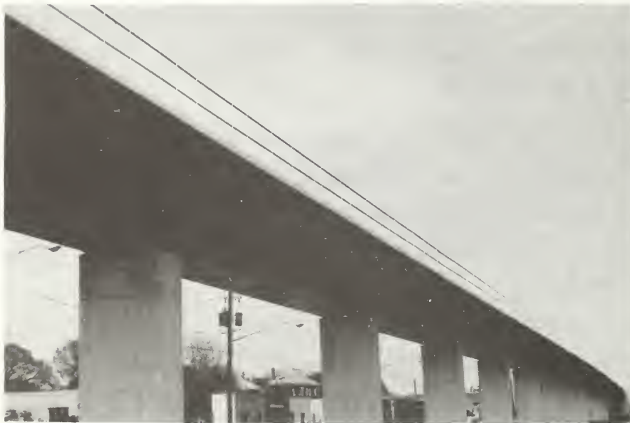
FIG. B.2. MARTA STRUCTURE NEAR SPRUCE STREET, AS SEEN FROM SOUTH SIDE. NOTE HANDRAIL, BUT NO NOISE BARRIER.
