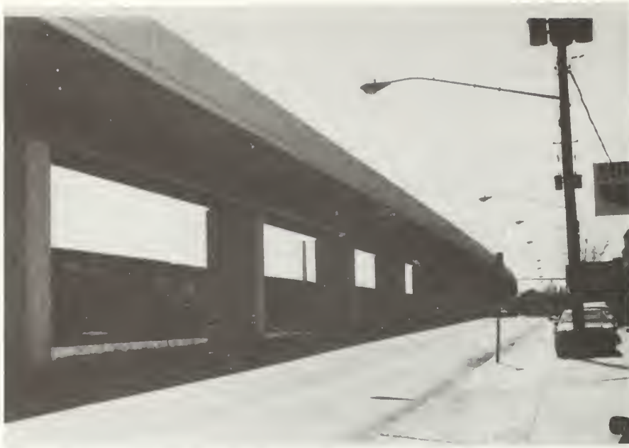
FIG. B.1. MARTA STRUCTURE NEAR SPRUCE STREET, AS SEEN FROM NORTH SIDE. NOTE NOISE BARRIER.
