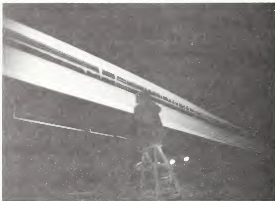
FIGURE 24. INSPECTING CLEAR INVERTED POWER RAILS AND GUIDANCE/AUXILIARY TRACTION SURFACE OF HEATED SECTION, WHILE SNOW AND ICE REMAINS ON SIDE-MOUNTED SECTION TO THE RIGHT
