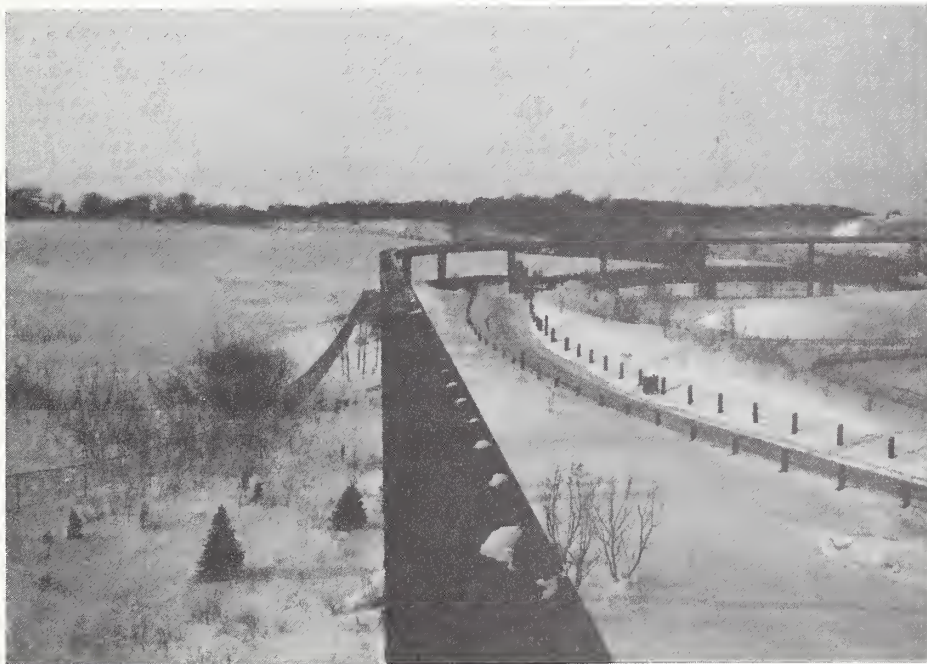
FIGURE 5. WIND FREQUENTLY CLEARS SNOW FROM GUIDEWAY
