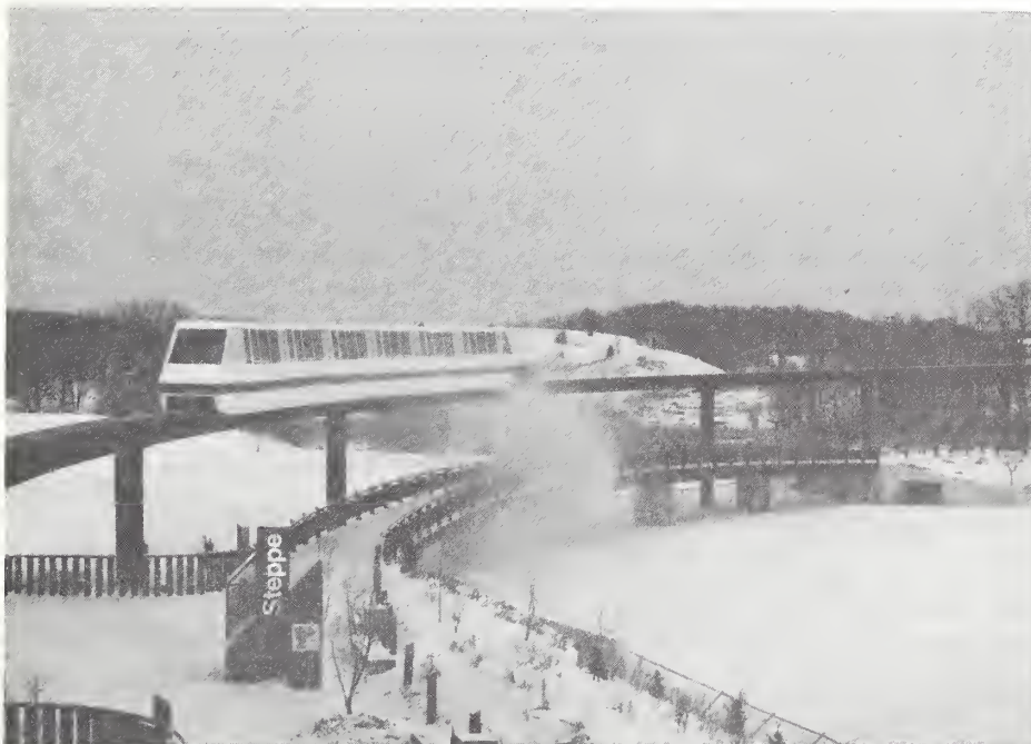
FIGURE 7. CLEAR GUIDEWAY AFTER SINGLE BRUSHING OF OVERNIGHT SNOWFALL
