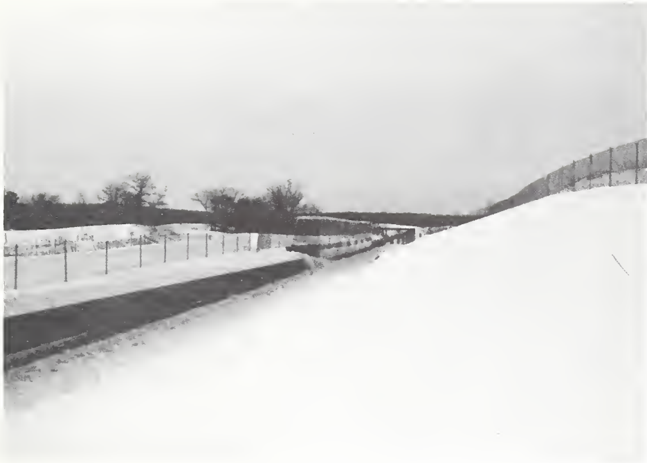
FIGURE 15. REMOVING SNOW, OVER 20 INCHES DEEP, THAT HAD BEEN PLACED BY A SNOWTHROWER
