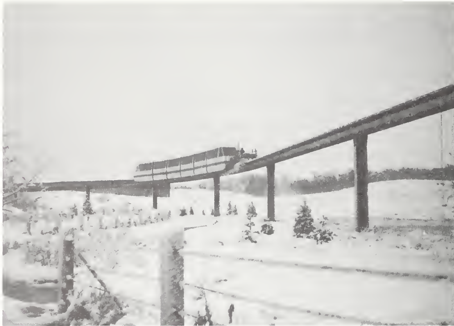
FIGURE 29. SNOW REMOVAL USING INTERIM MAINTENANCE SUPPORT VEHICLE CAPABILITIES
