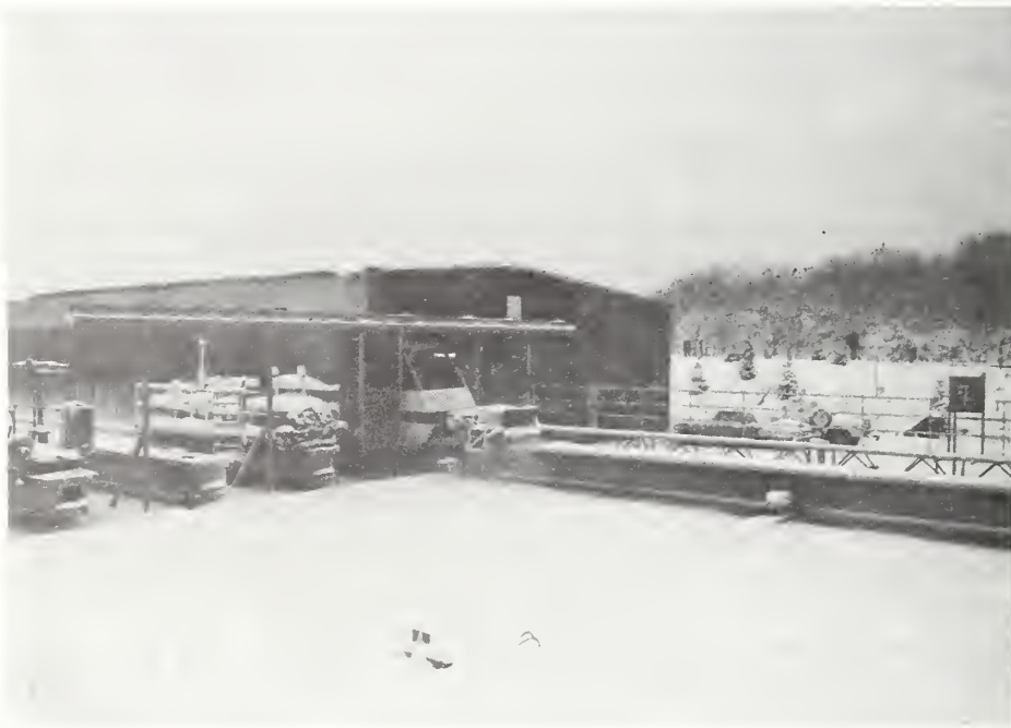
FIGURE 18. TRAIN EXITING MAINTENANCE BUILDING WHILE REMOVING SNOW FROM THE TRANSFER BEAM
