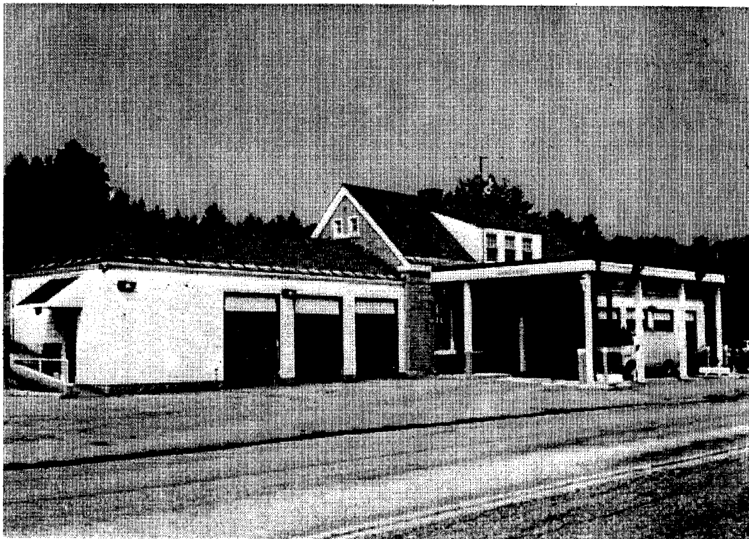
North Troy: Primary inspection egress and administration building
