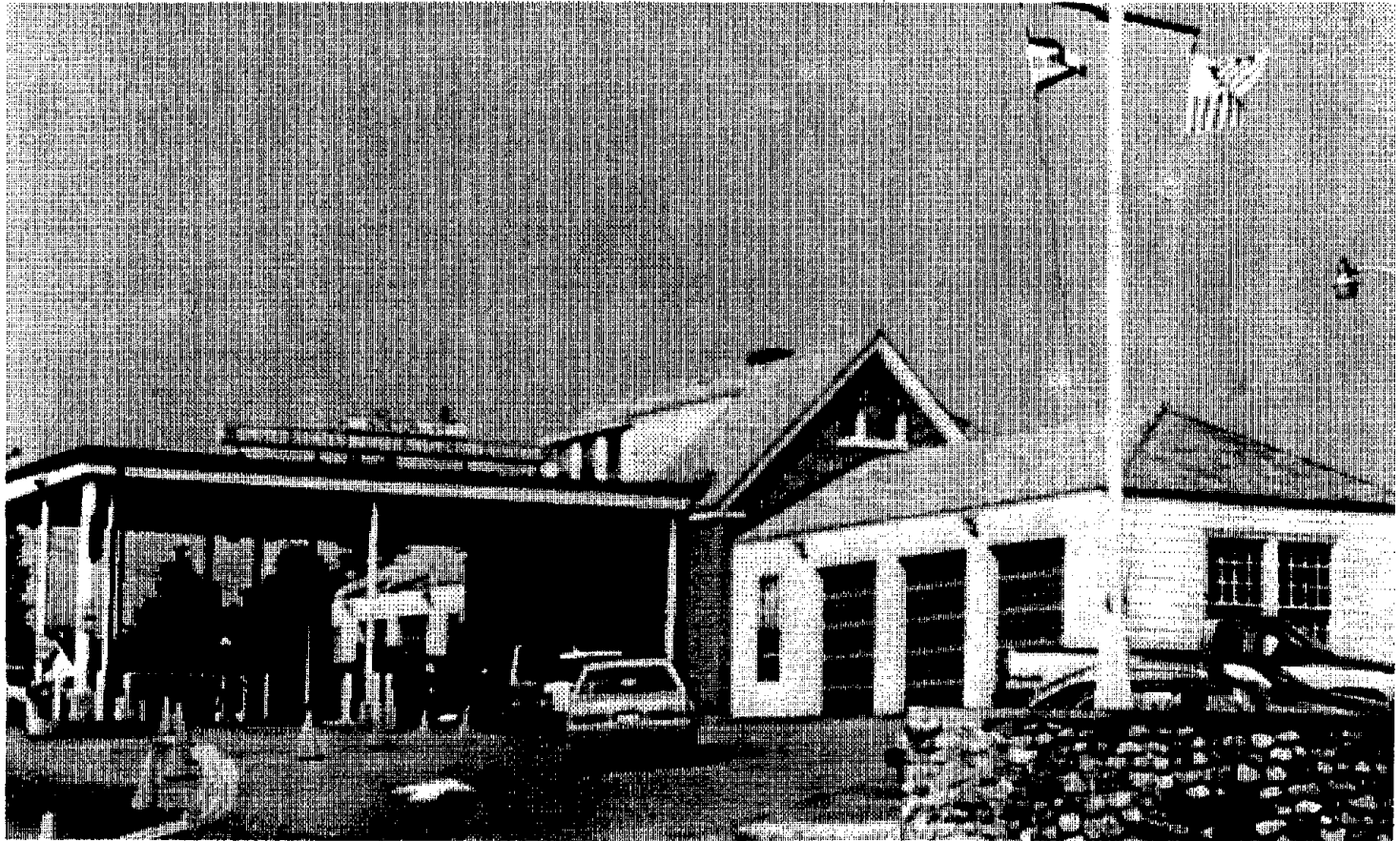
Norton: Administration building and primary inspection lanes
