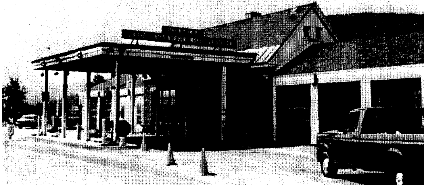
Canaan: Administration building and primary inspection lanes
