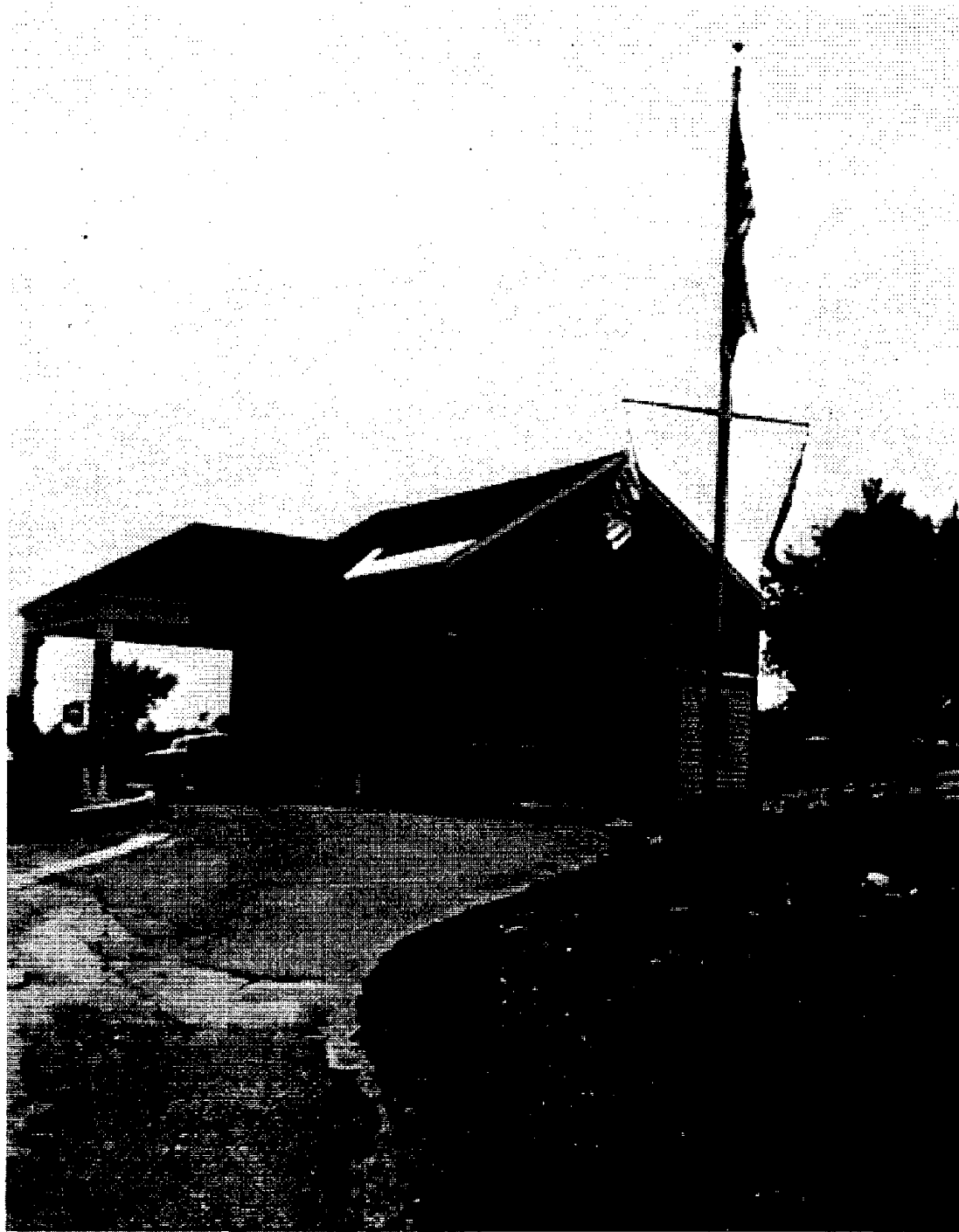
Alburg Springs: Approach to inspection station and administration building
