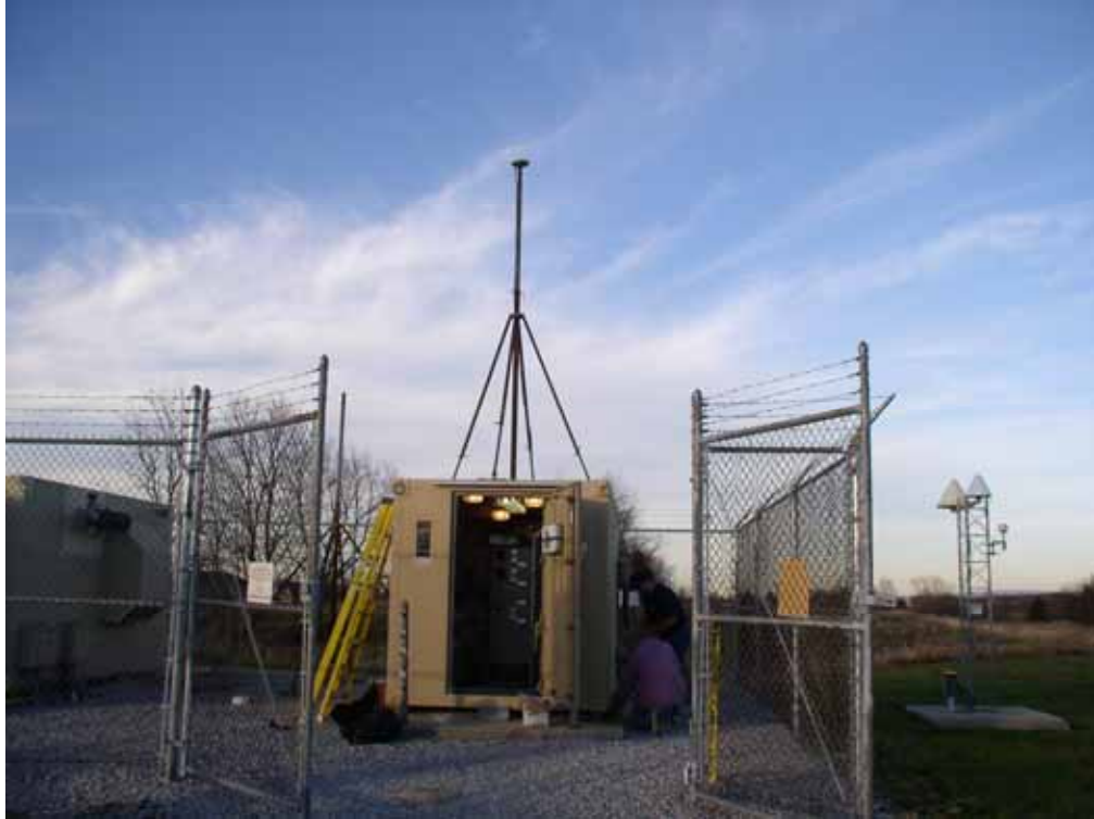
Figure 24. The Hagerstown GWEN site with a pentapod marine antenna 4 to 5 meters above the hut to search for the cleanest signals.
