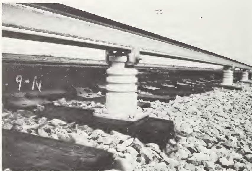
FIGURE 13 CONTACT RAIL INSTALLED ON WOOD TIES
