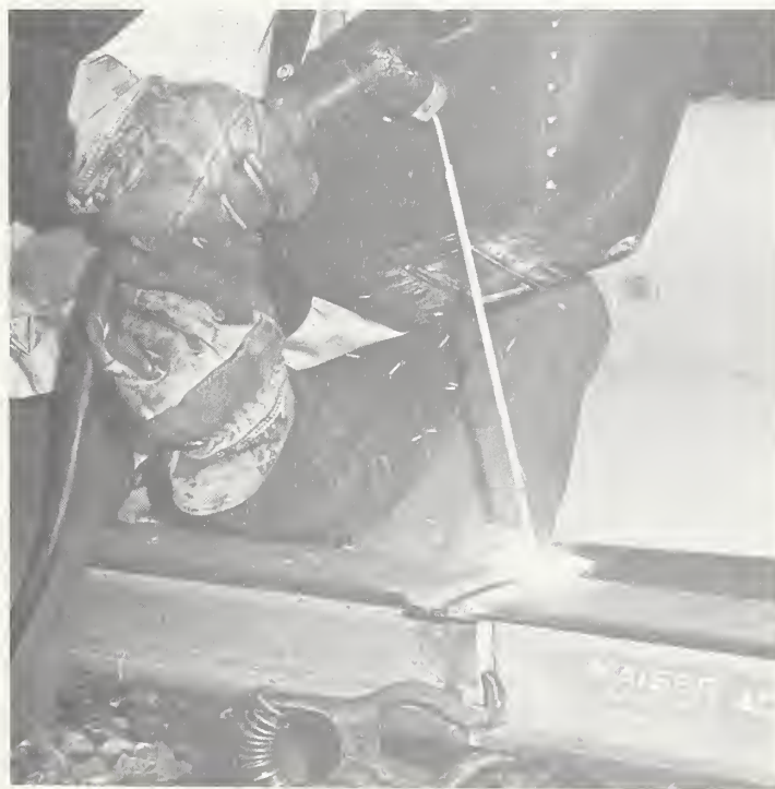
FIGURE 8 WELDING STEEL PORTION OF COMPOSITE RAIL
