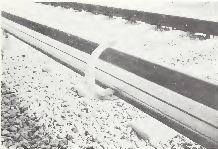
FIGURE 14 COVER BOARD BRACKET
