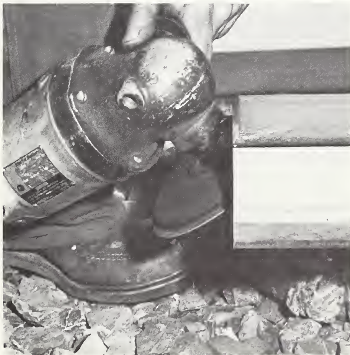
FIGURE 4 GRINDING RAIL ENDS PRIOR TO WELDING
