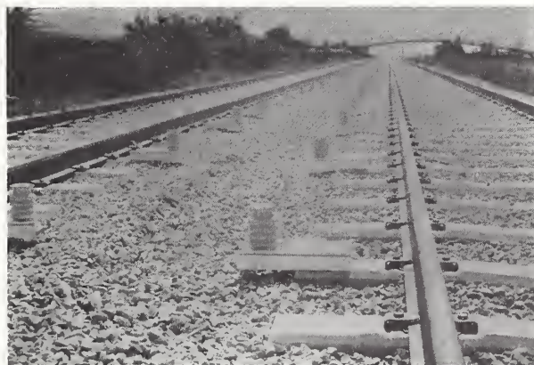
FIGURE 12 INSULATOR INSTALLATION-CONCRETE TIE SECTION
