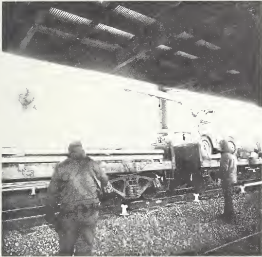
FIGURE 1 OFF-LOADING OF TRANSDUCTOR™ RAIL
