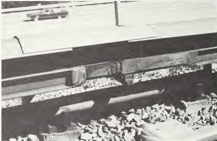
FIGURE 7 TYPICAL INSTALLATION OF EXPANSION JOINT
