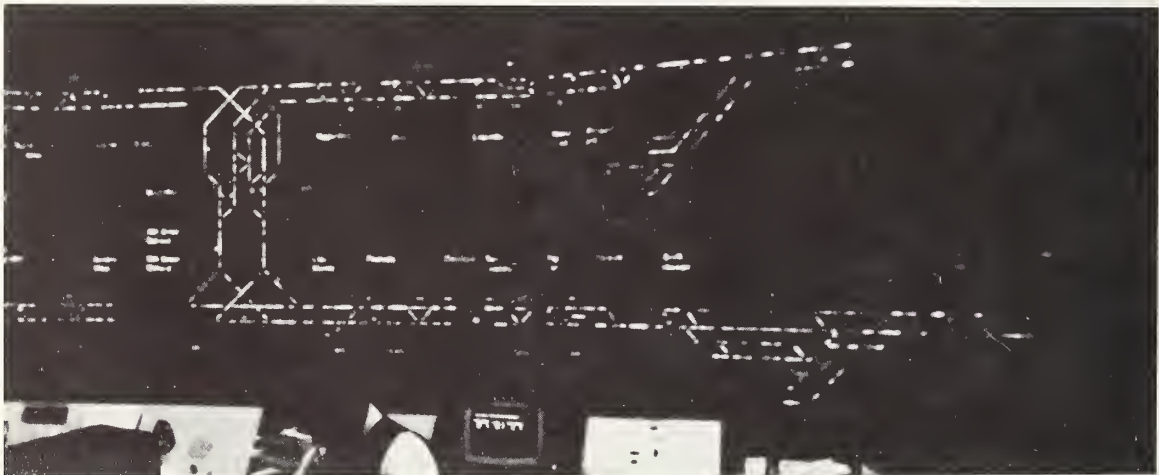
Technicians at underground BART control system monitor all train movements, identified on wall-mounted console. The Speno grinding train was used to remove mill scale from track, to assure proper electrical contact needed for this display.
