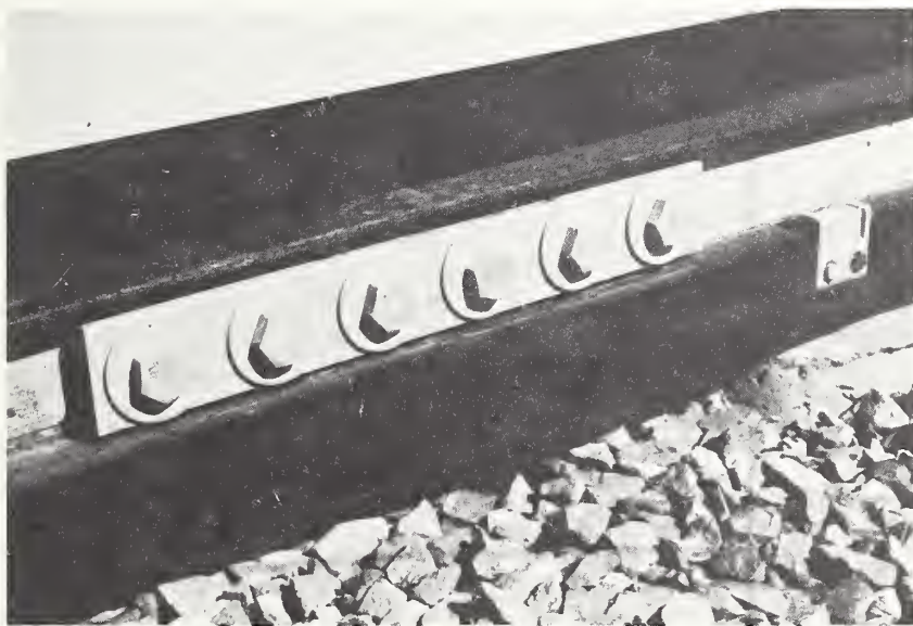
FIGURE 3 BOLTED JOINT
