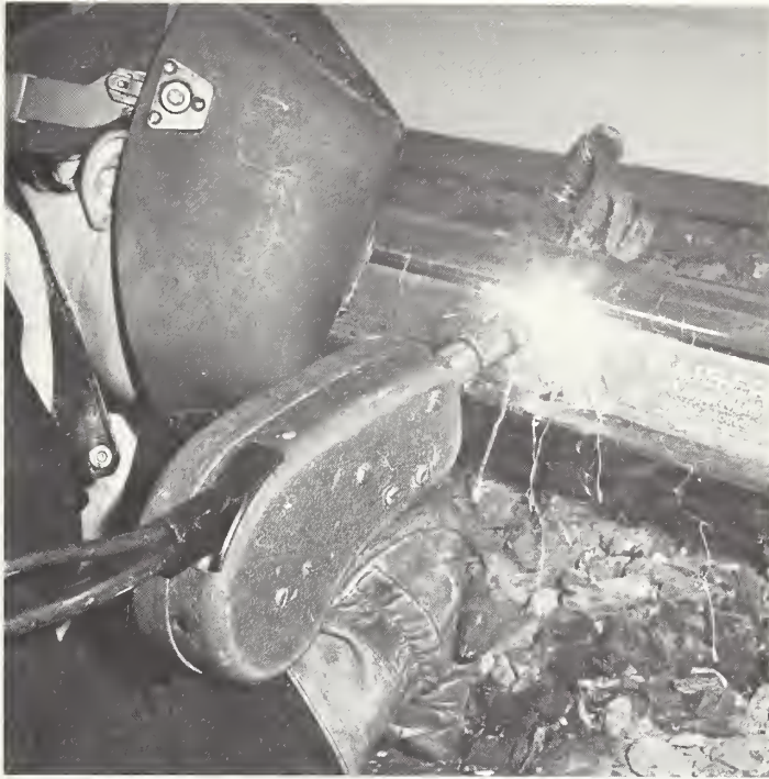
FIGURE 11 WELDING ALUMINUM PORTION OF COMPOSITE RAIL WITH MIG GUN
