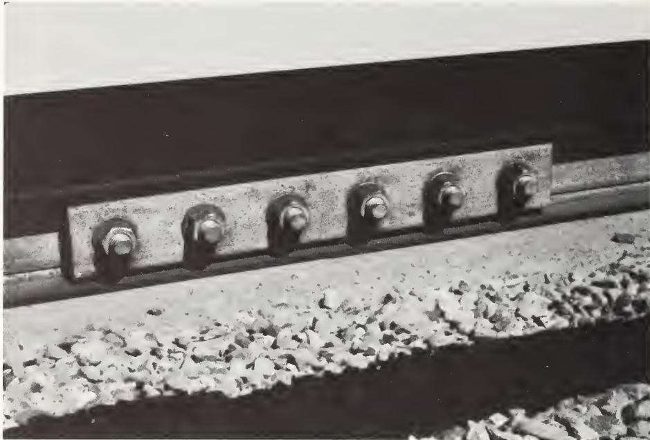
FIGURE 4 BOLTED JOINT
