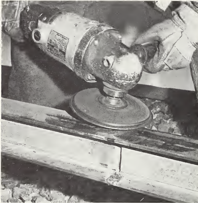
FIGURE 9 GRINDING STEEL SURFACE SMOOTH ON TOP OF RAIL
