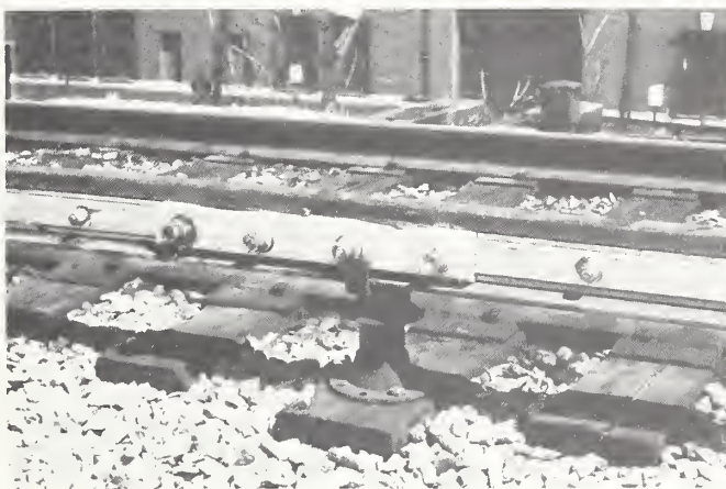
FIGURE 11 COMPOSITE THIRD RAIL JOINT
