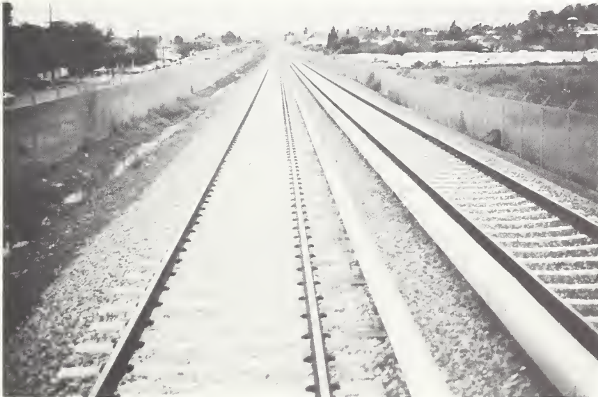
FIGURE 31 TRACK AFTER COMPLETION OF MAINTENANCE
