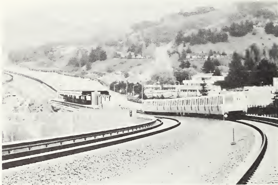
FIGURE 32 CURVE AT ORINDA
