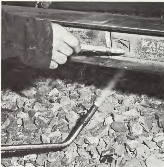
FIGURE 9 GRINDING STEEL SURFACE SMOOTH ON TOP OF RAIL
