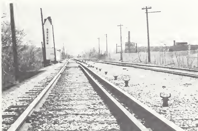
FIGURE 12 INSTALLATION IN PROGRESS
