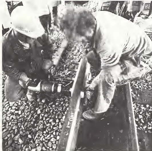
FIGURE 3 INSTALLATION OF HUCK BOLT THROUGH SPLICE JOINT
