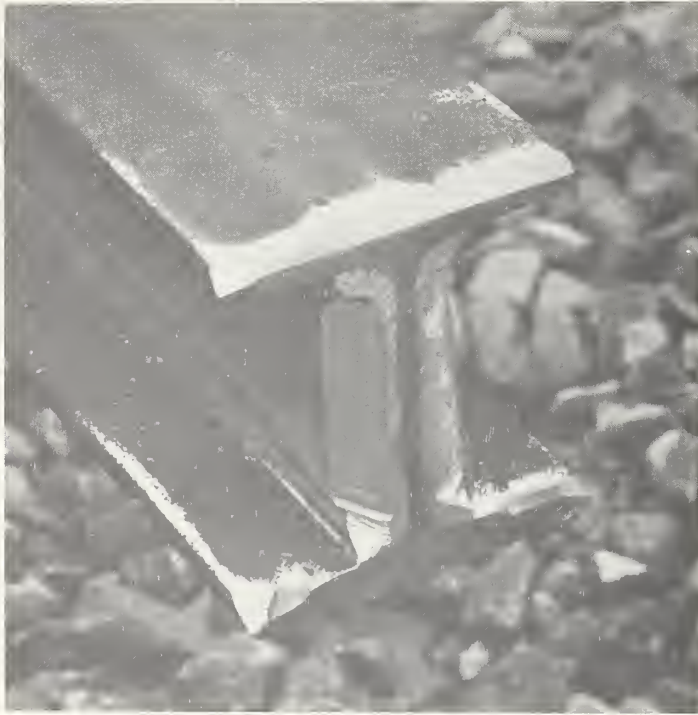
FIGURE 5 RAIL END PREPARED FOR WELDING
