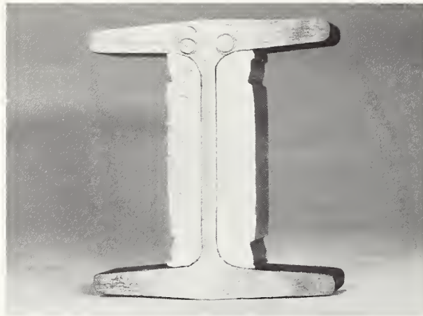
FIGURE 22 SECTION THROUGH WORN THIRD RAIL
