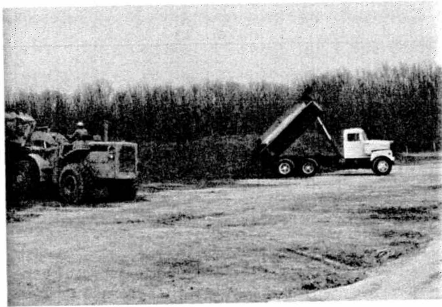
Figure 15 Stockpile of reclaim at MHTD lot.
