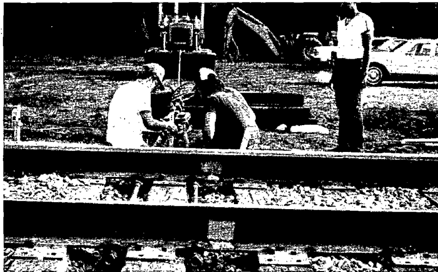
PHOTO. 6 - APPARATUS FOR SETTING INITIAL IMPERFECTION AND MEASUREMENT OF LATERAL RESISTANCE
