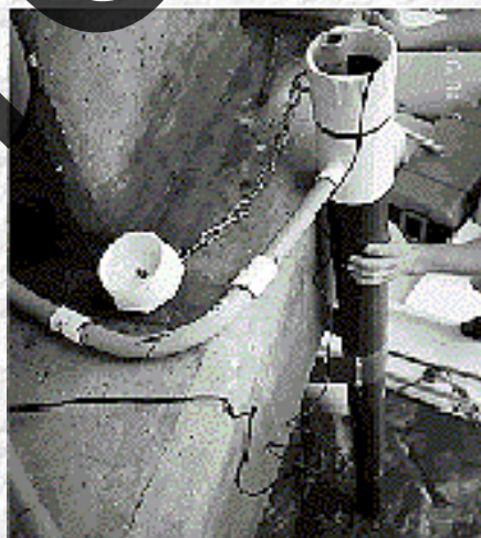
Figure F-1. Sonic Instrument on Johns Pass Bridge, Florida
