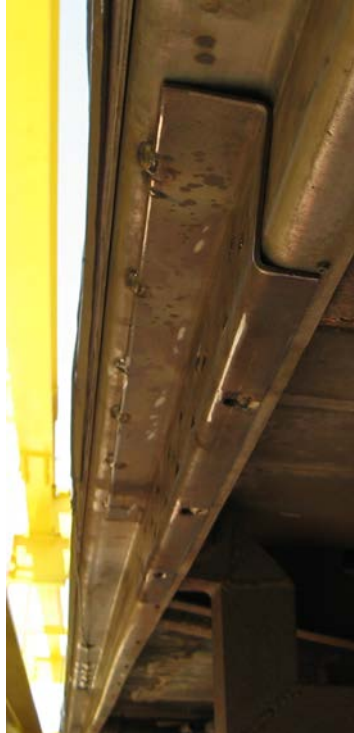
Figure 6. Patch Installed on Car 244 Side Sill
