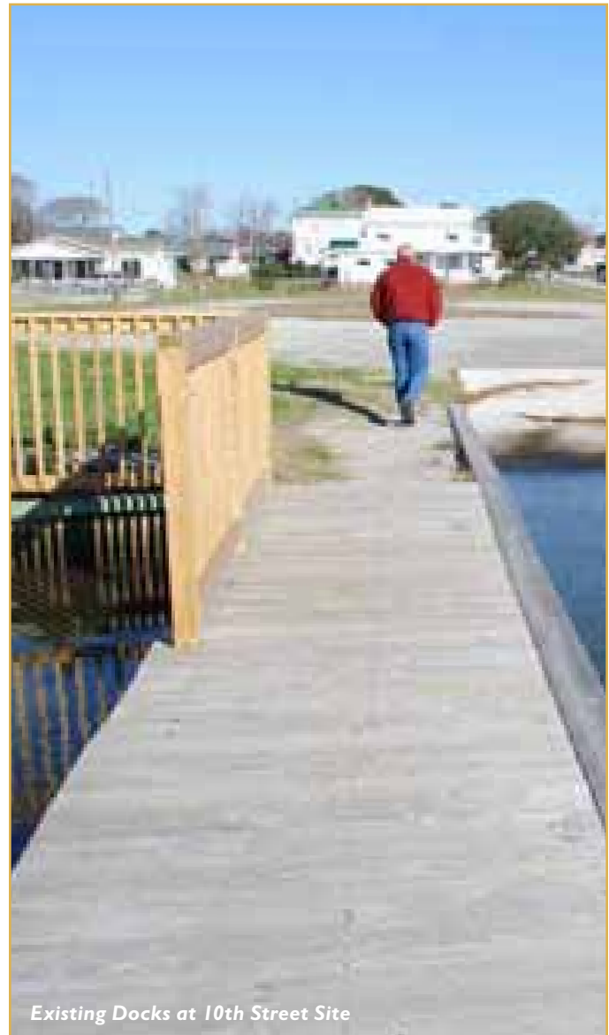
Existing Pier at 10th Street Site
