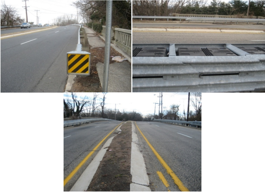
Figure 4. Photos of NJ route 71
