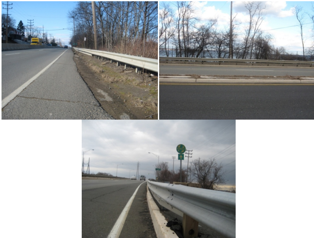
Figure 3. Photos of NJ route 35
