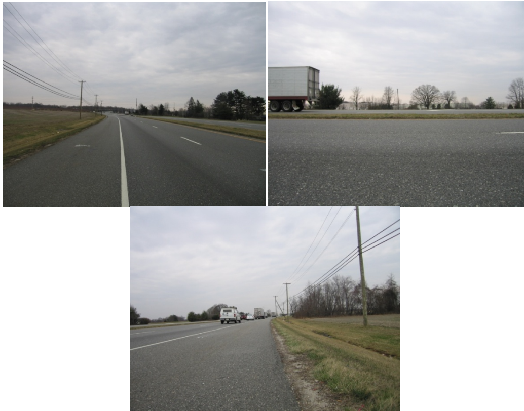
Figure 6. Photos of NJ route 322
