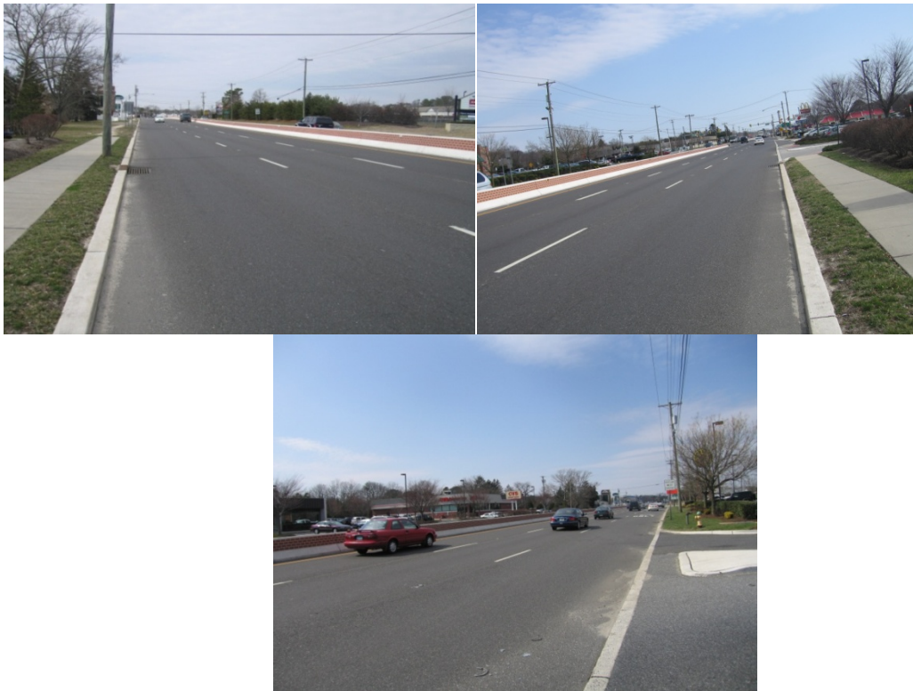
Figure 1. Photos of NJ route 30
